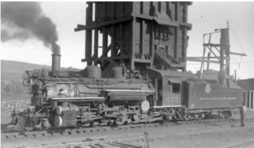
Figure 15 - West Side in 1939 showing Equipment Shelter Otto Perry photo from Denver Public Library
