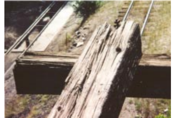
Figure 13 - Timber Connection on East Side
