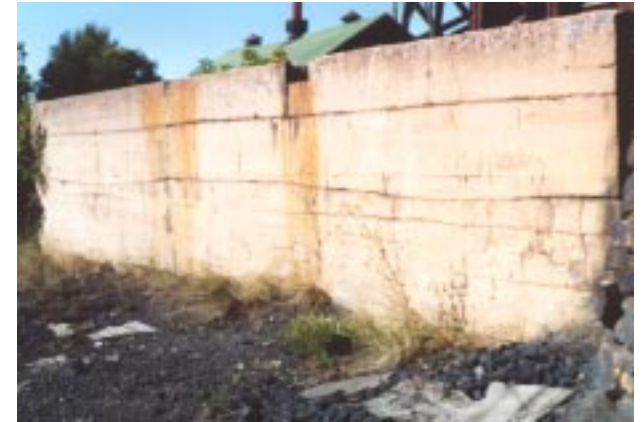
Figure 14 - East Wall of Coal Hopper
